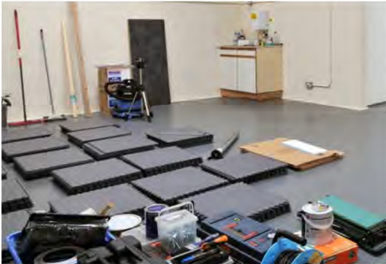
Break down the pallets and allow tiles to acclimatise
