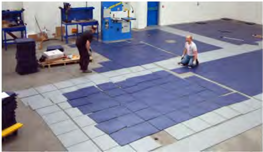
Split the pallet and spread the tiles across the floor prior to starting installation.
